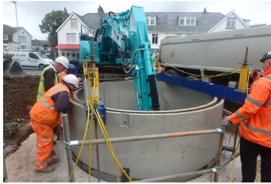
ix. Lowering shaft for housing pumping station
